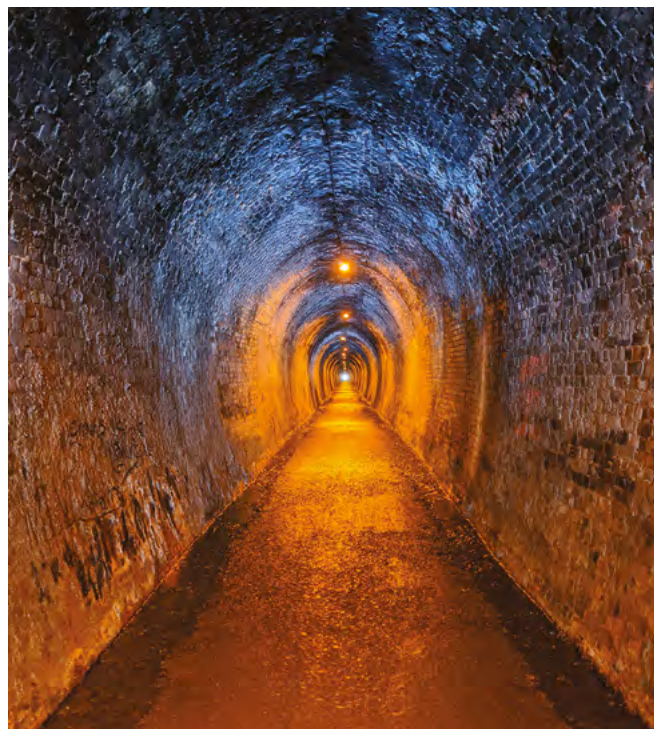
PHOTO: KARANGAHAKE GORGE TUNNEL PHOTOGRAPHY: EDD / ADOBE STOCK
